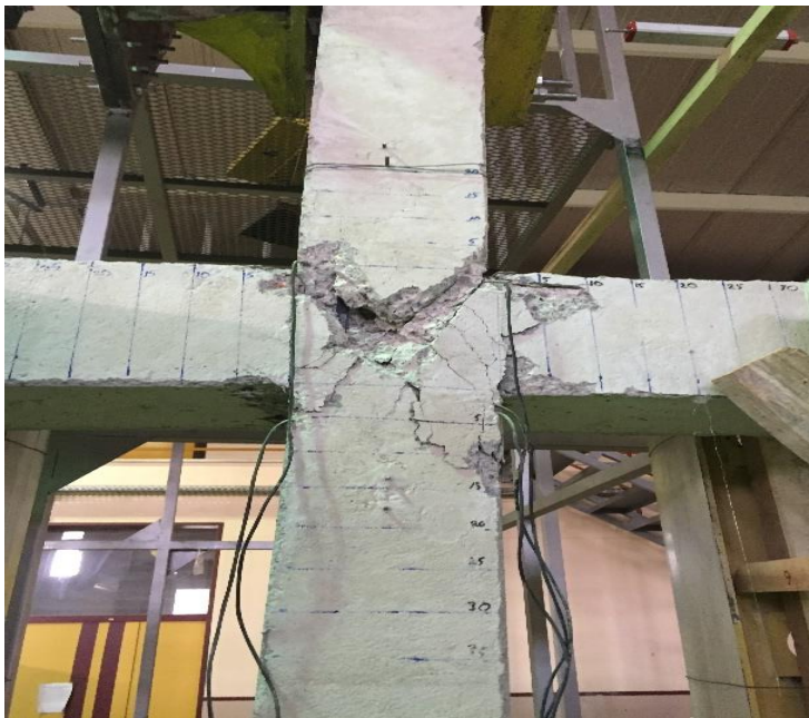
Figure 14. Crack development in SAMPLE 2
