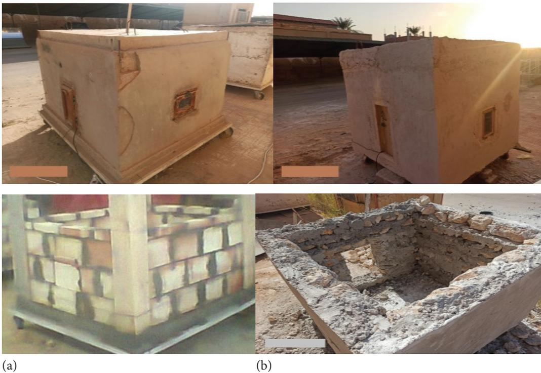
**Figure 2.** Construction process of the cubicles (a) hollow brick (b) local stone.
