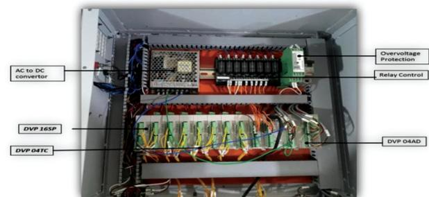
Figure 6. Construction layout of hardware in NMDAS.
