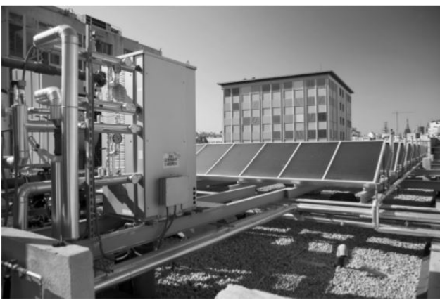
Figure 1. Cogeneration cycle with flat plate collector.
