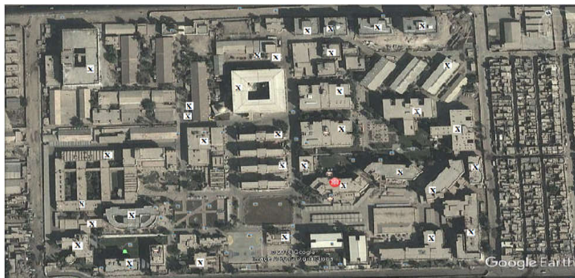
Figure 1. University of Technology from the air illustrating the location of operating generators
