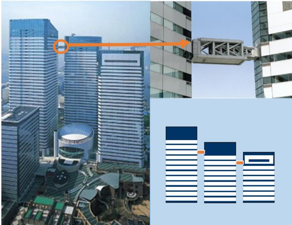
Figure 1. Harumi Island Triton Square Office Tower [4].
