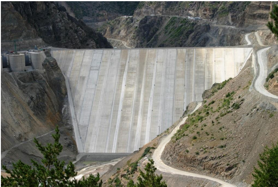
Figure 2. Torul CFR Dam.
