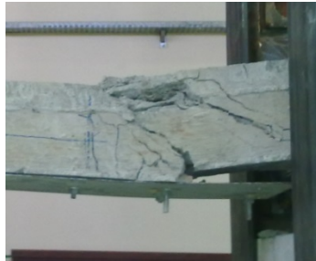
Figure 13. Pull-out of bolts at near support [19]
