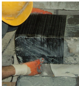
Figure 7. Application of CFRP sheets at support sections [19]
