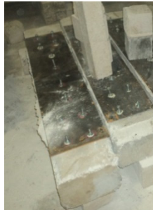
Figure 5. Member strengthened with steel plate [19]
