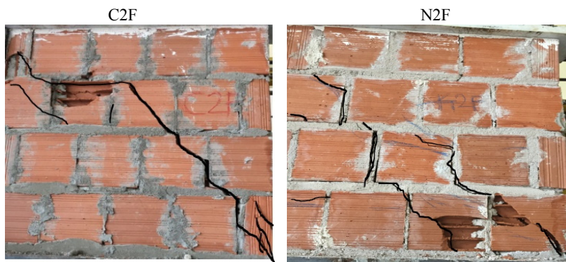
Figure 6. Damage of the Walls produced with Fabricated Brick
