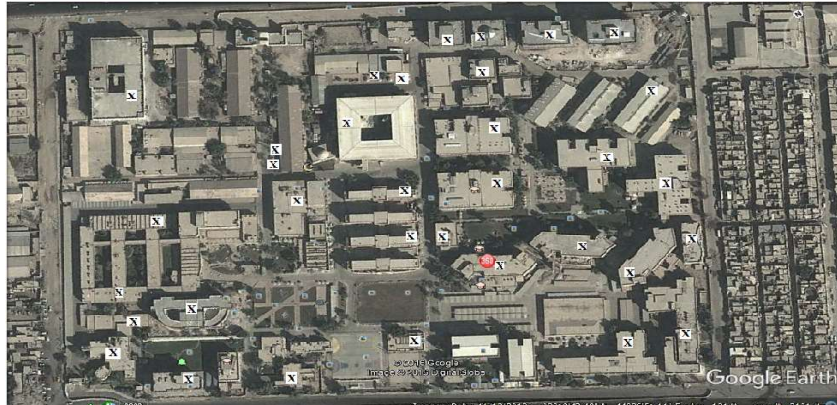
Figure 1. University of Technology from the air illustrating the location of operating generators
