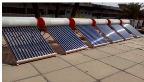
Figure 2. Solar water heater system for ERET
