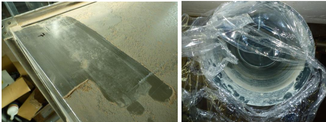
Figure 1. Sample contamination during ducts assembly (on the outside – left, on the inside - right)
