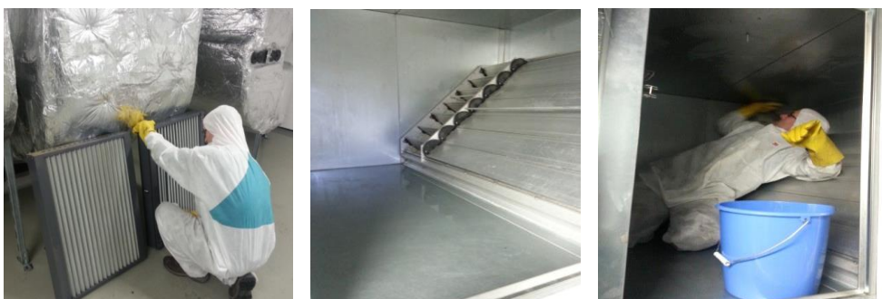
Figure 11. Sample of typical examples of wet cleaning (left droplet eliminator, right filter chamber)
