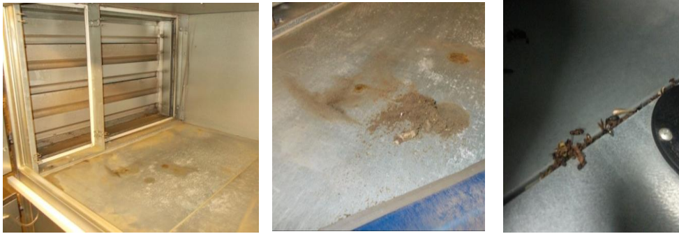
Figure 9. Demonstration of pollution of the filter chamber on the side of the intake of fresh air (left), solids trapped in the joint between the panels (right)
